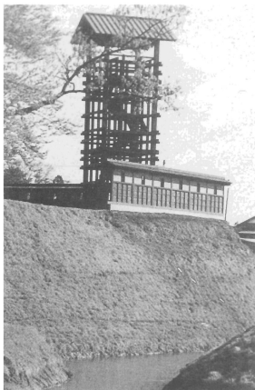
A section of wall and the openwork observation tower from the reconstructed castle of Sakasai. The grassy bank slopes steeply down to a wet moat. This tower would have been typical of castles of this size, and provided the distant outlook later to be supplied by the tower keep. (Photograph by courtesy of Sakasai-chō Board of Education)
