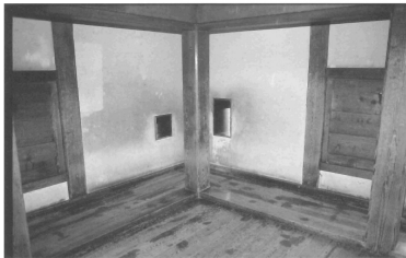
The interior of the keep of Matsumoto, built in 1597, gives a good impression of the inside of a late Sengoku castle. The construction is entirely of wood, with plastered walls across a narrow walkway from the central room. The windows are fitted with heavy wooden shutters and there are small defensive ports for arrows or guns.
